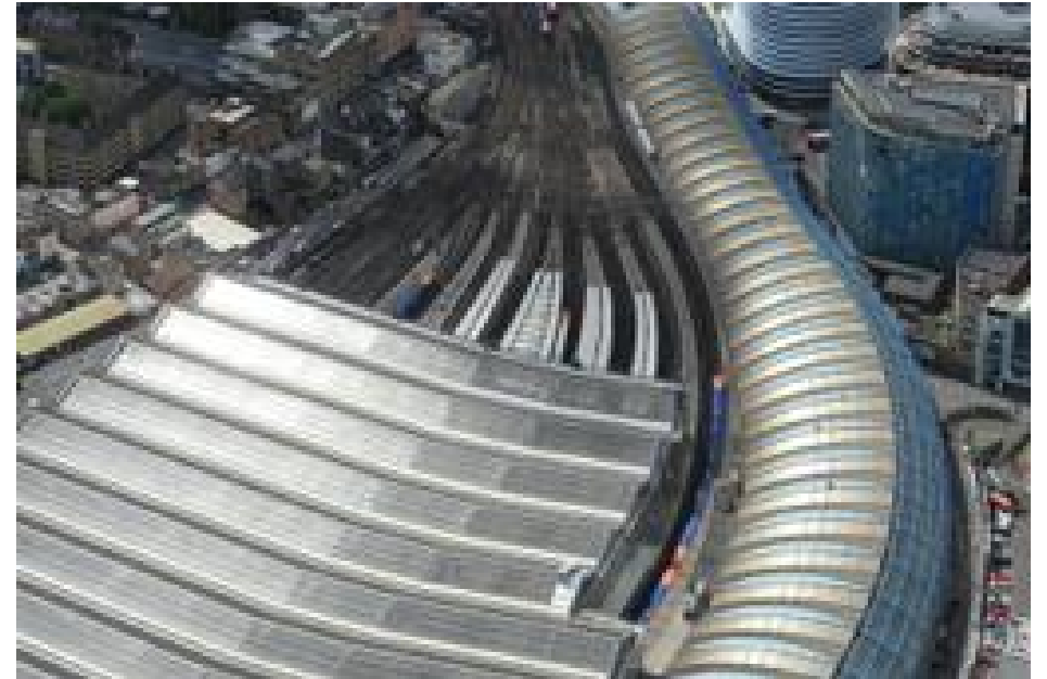
London Waterloo station
