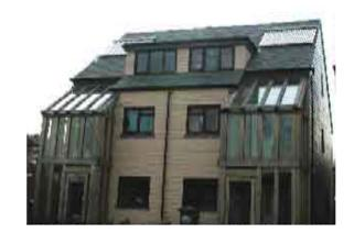
3.8.6 New homes on Portswood Road. Southampton (Hvde Housing Association) with direct solar power from photovoltaic cells and passive solar heating via fenestration
