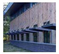
• Redirecting daylight with light shelves, prismatic glazing and other reflective systems can extend naturally lit interior space to 10 -11m deep.
