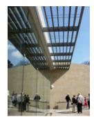
Fig 3.6 brise soleil solar shading
