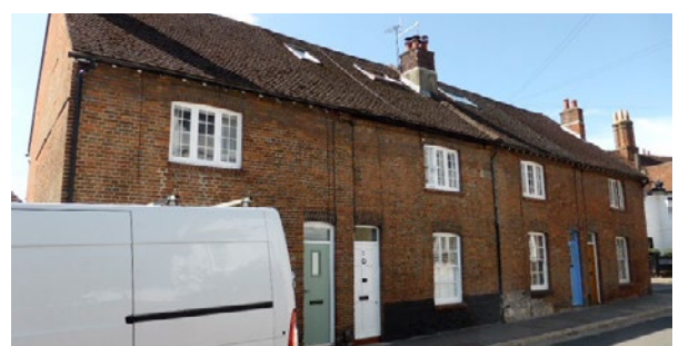
1 to 4 Purbrook Cottages
