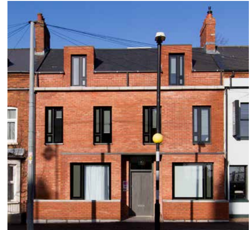
Sensitive infill development evolves the existing character by reflecting the façade composition and fenestration of adjacent homes, but introducing a contemporary design interpretation. Home for RVH, Belfast. (Image credit: Aidan McGrath).
