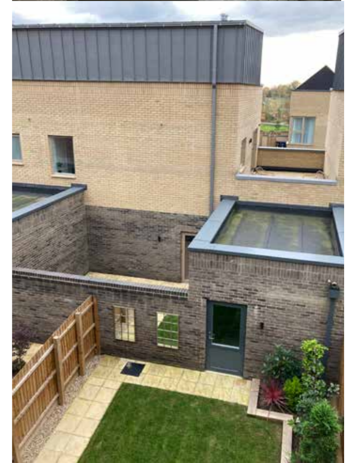
Access to smaller balconies and outdoor space from bedrooms to the front of homes, with smaller private gardens to the rear at Waterbeach, Cambridge.
