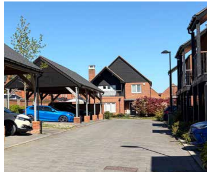
Parking Courts as part of public realm by front entrances of adjacent development at Barton Farm, Winchester.
