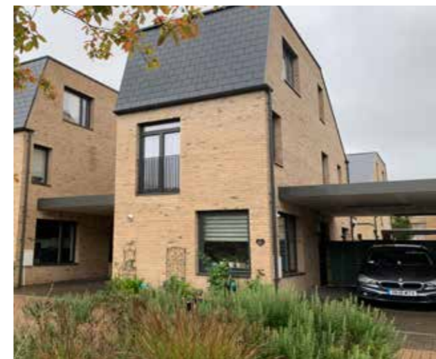
Car ports are carefully integrated between homes on-plot, in Barton Park, Oxford.
