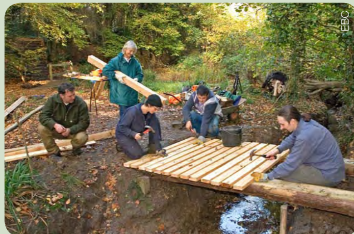
The BTCV NVQ field team built a new bridge over the stream at West End Copse. The project used timber grown at Itchen Valley Country Park felled as part of a woodland improvement scheme and converted into planks
